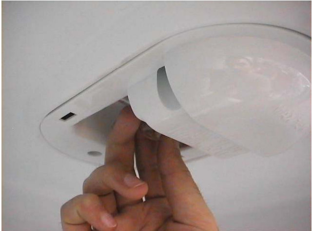
Loosen the lamp and replace it.
